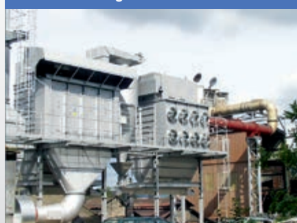
Flat-tube heat exchanger without cooling air recirculation
